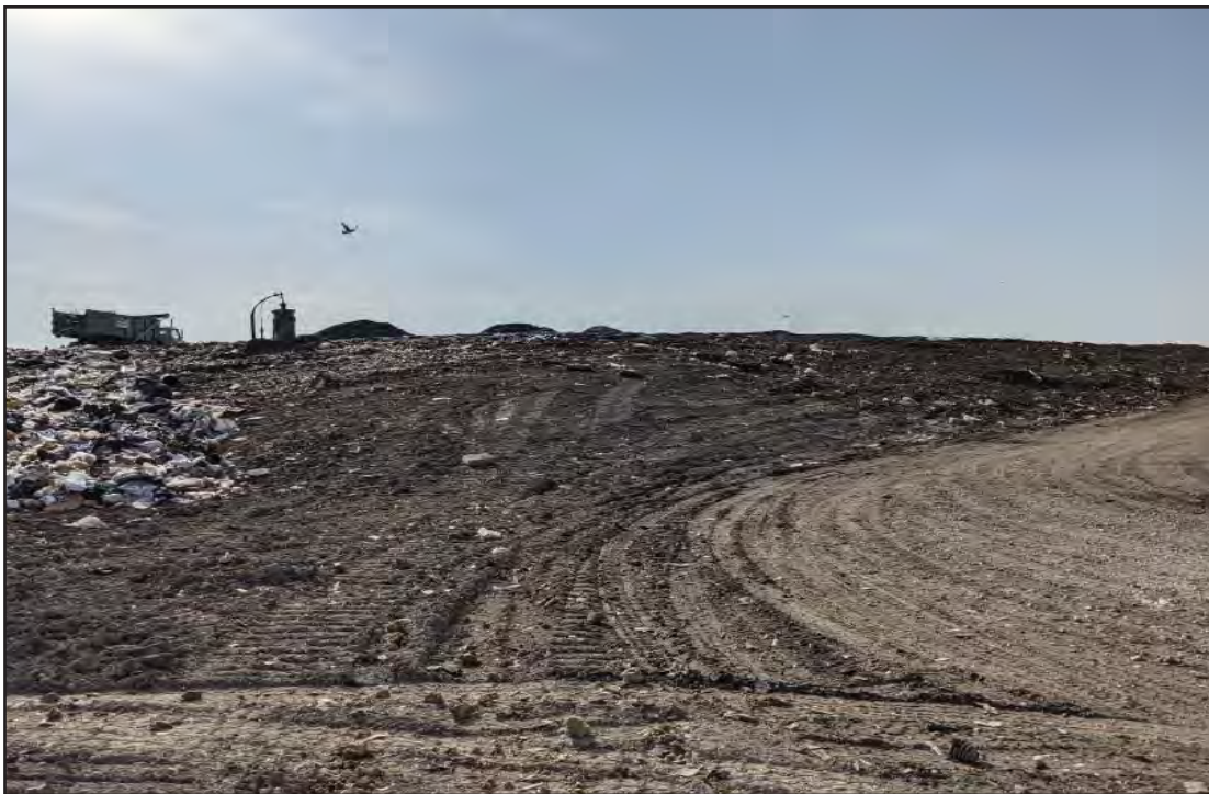
current lift, covered with soil on outboard slopes and access road
