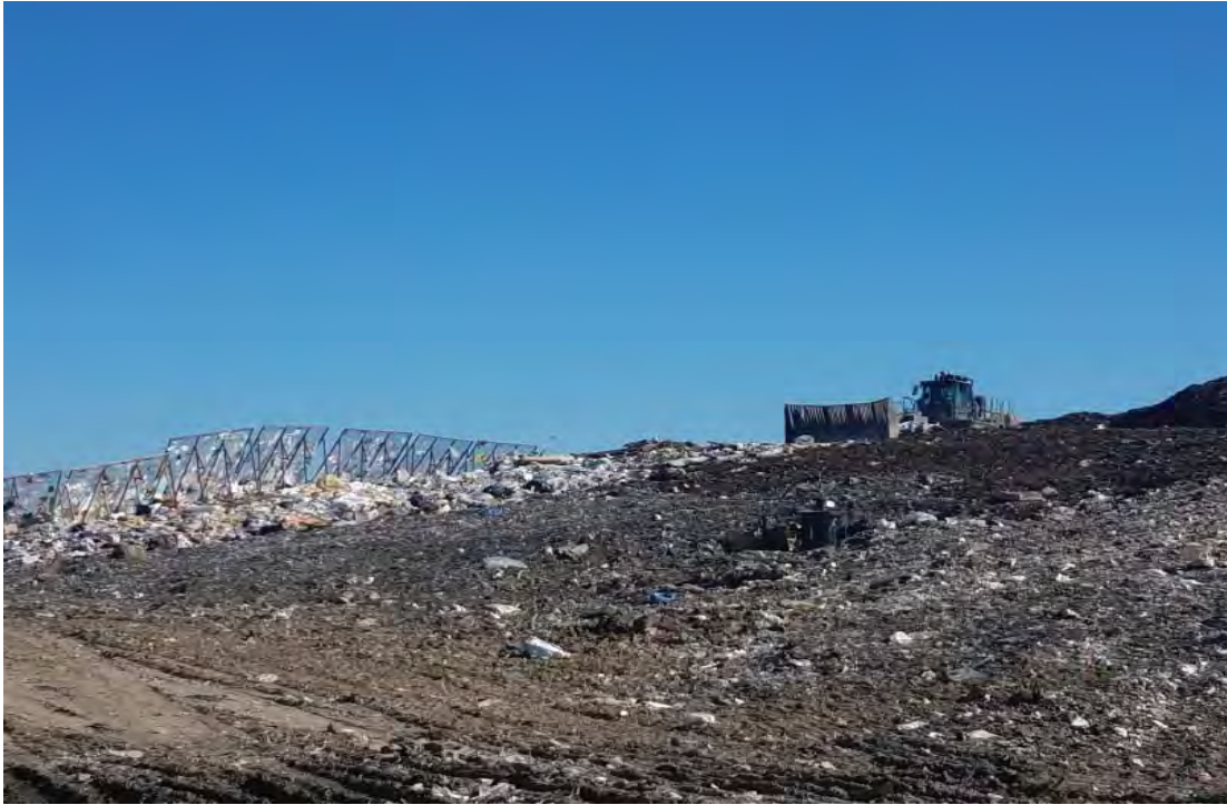
Working face with mobile fencing to catch litter on a high wind day
