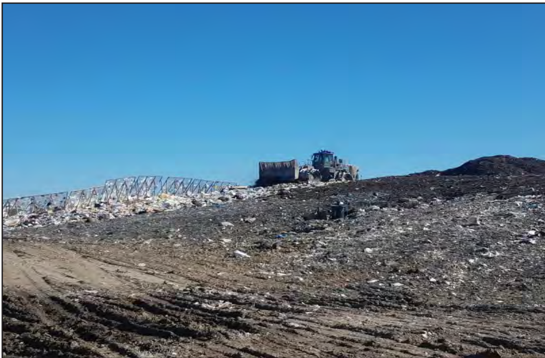
Working face at East edge of Phase 7, bare edge of slope.
