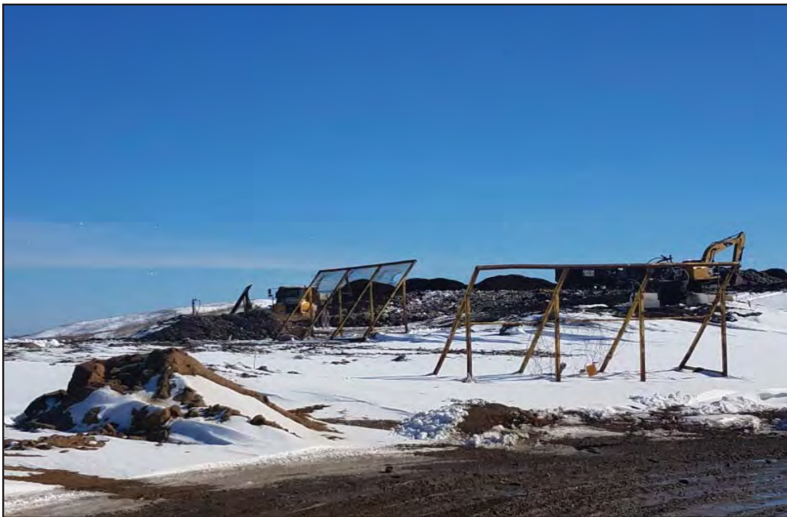
Tipping of trucks in Southeast corner of Phase 7 North
