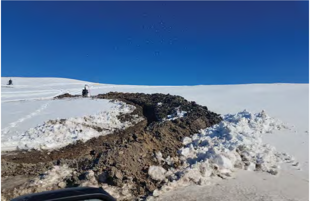
Repair to connections between wells to insure gas containment
