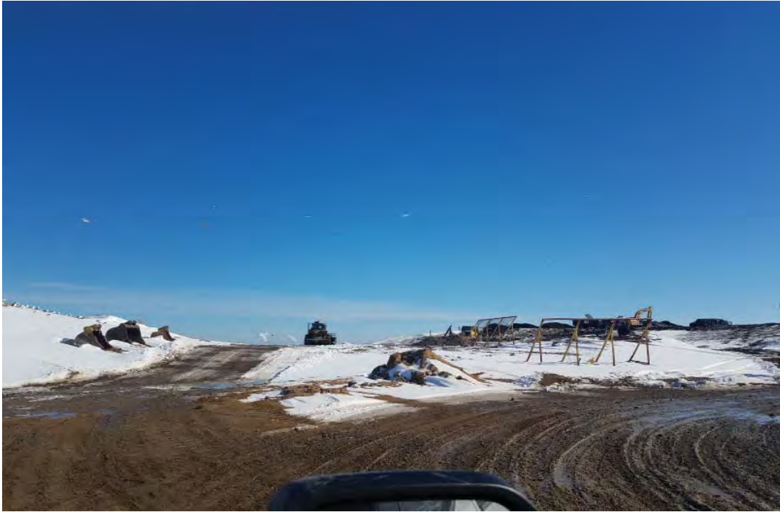
Phase 7 viewed from the Northwest, right hand road goes to working face; left hand road allows access of staff to LFG management wells
